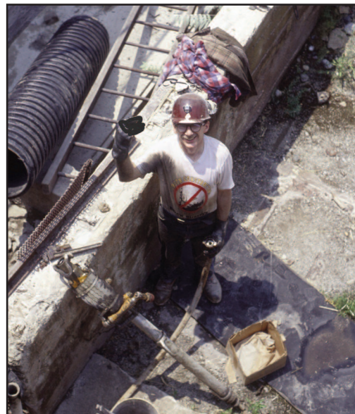
John Kolic working at the site of the Great Sterling Mill.
