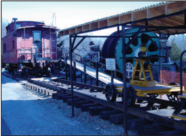
Newly installed railroad track connecting our caboose and the new pavilion may be used for running the smaller motorized units and handcar on special occasions.
