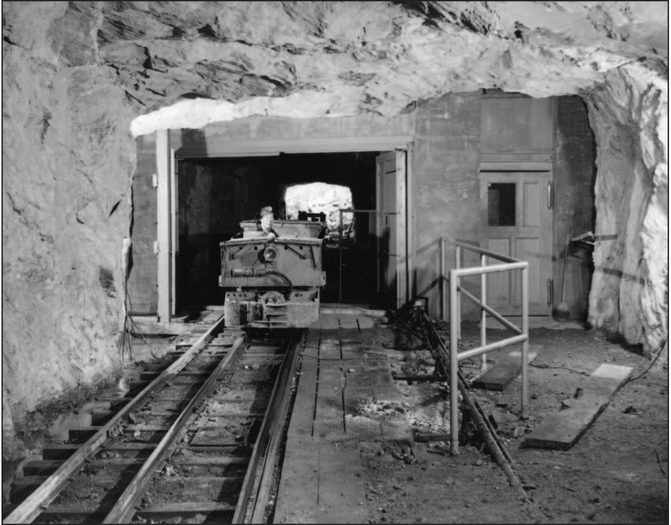
This photograph from the mid 1950s shows part of the new shaft development -- the doors leading out of the adit into the lower yard. Blasted material in the lower yard can be seen in the background. Rock (not ore) was being blasted in the lower yard to make it level for the train tracks. This rock was trammed into the adit, dumped onto the grizzly rail, diverted below, then used for filling stopes and pillars throughout the mine.
