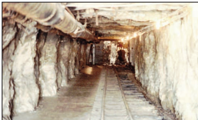
The adit level, as found in 1989 upon re-entry to the mine.
