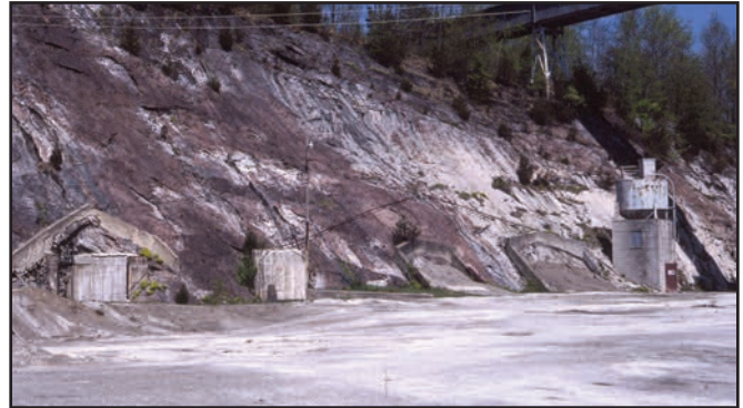
Sealed adit entrance and safety exit, as they appeared when the property was purchased in 1989.
