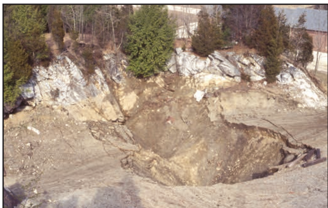
Subsidence in the Fill Quarry.
