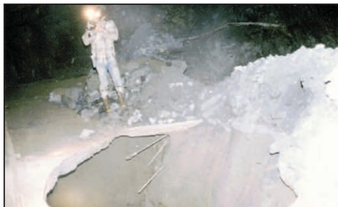
Subsidence on the 700 level, being filmed by Rich Luzzi.
