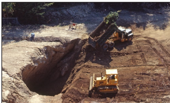
Filling in the subsidence hole in the Passaic Pit.
