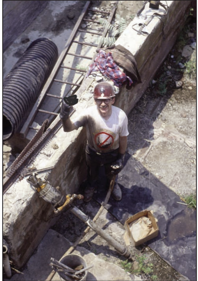
John Kolic working at the site of the Great Sterling Mill.
