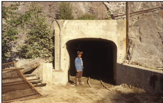
John Kolic standing at the adit after the concrete plug was totally removed.
